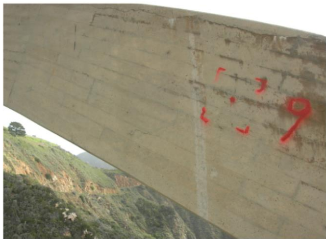
Spall on right arch, south end
